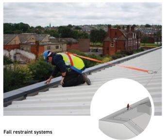
A standard fall restraint system is installed at 2,3 meters from the roof edge.
