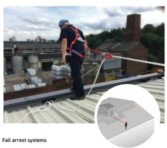
The design of a fall arrest system must always be supported by published calculations applicable to the roof structure in question. In addition, the height of the building and fall clearance must be considered.
